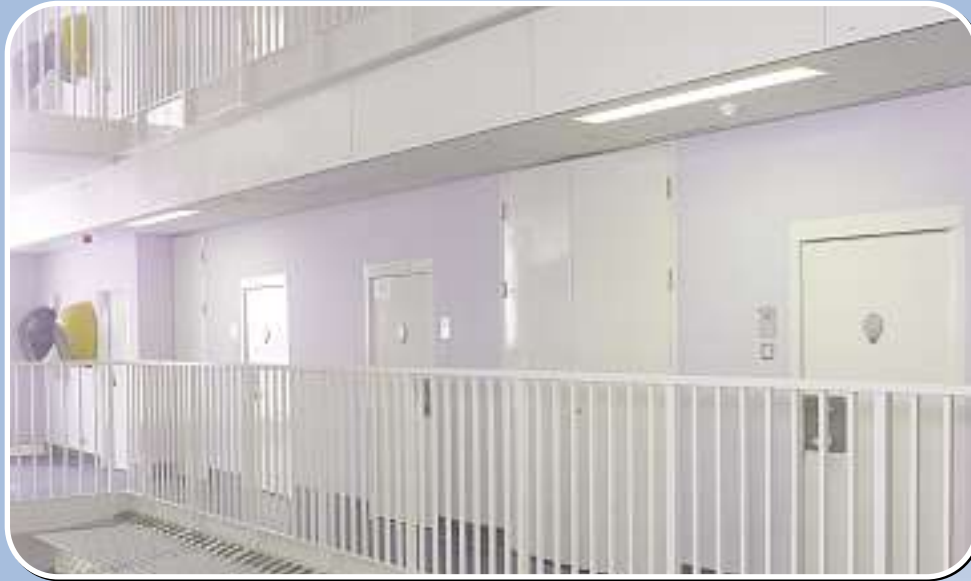
• Prison Wing Bulkhead Ducting, enclosing services into cells and incorporating lighting, smoke detection, sprinkler system, air plenum, and service access doors (detailed)
